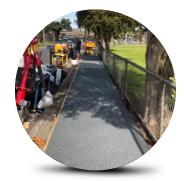
Permeable pavements, unlike conventional asphalt paving, allows water to pass through the surface, reducing storm water runoff and pollution in waterways.
